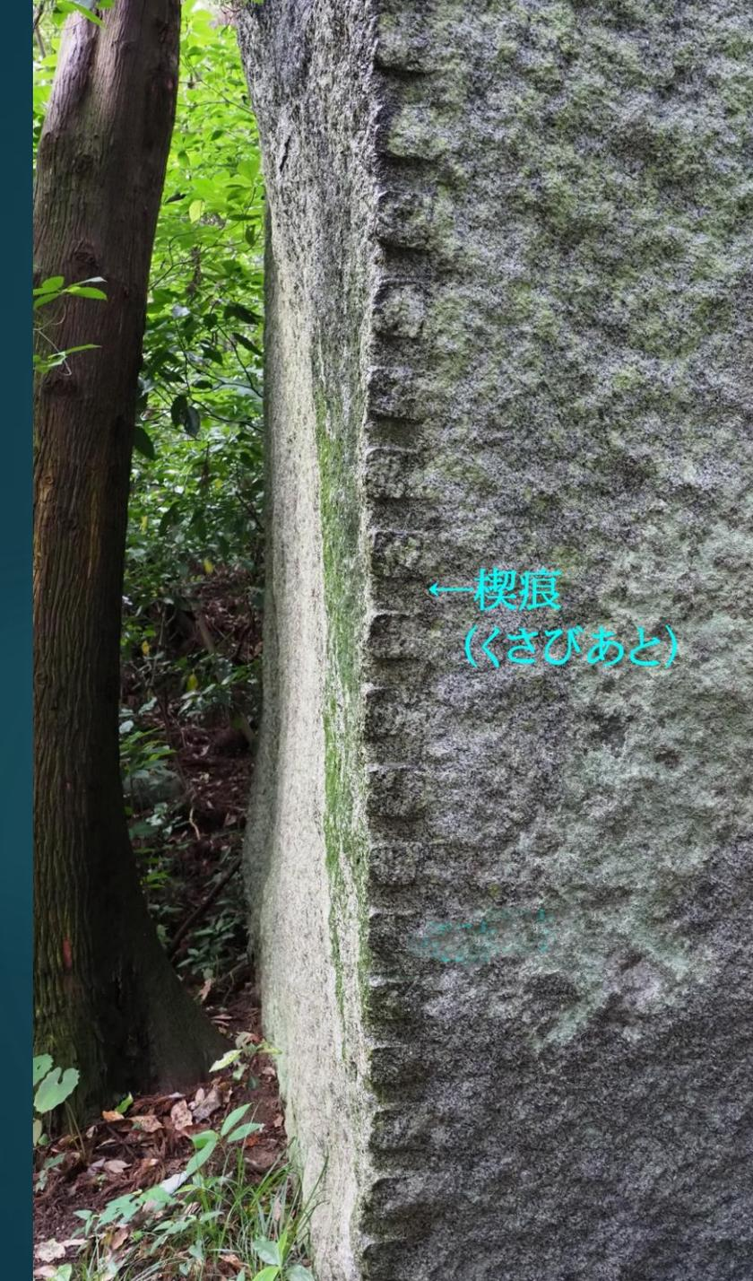
A close-up photograph of a stone wall. The wall is constructed from large, rectangular stones. A prominent vertical groove, known as a 'kuzabi' (wedge mark), runs down the center of the wall. The stone surface is covered in a layer of green moss. To the left, a tree trunk is visible, and the background is filled with lush green foliage.
